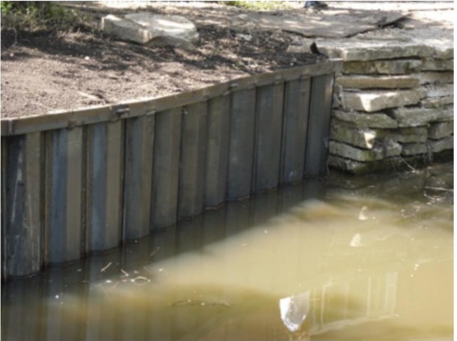
Example of an intact retaining wall
